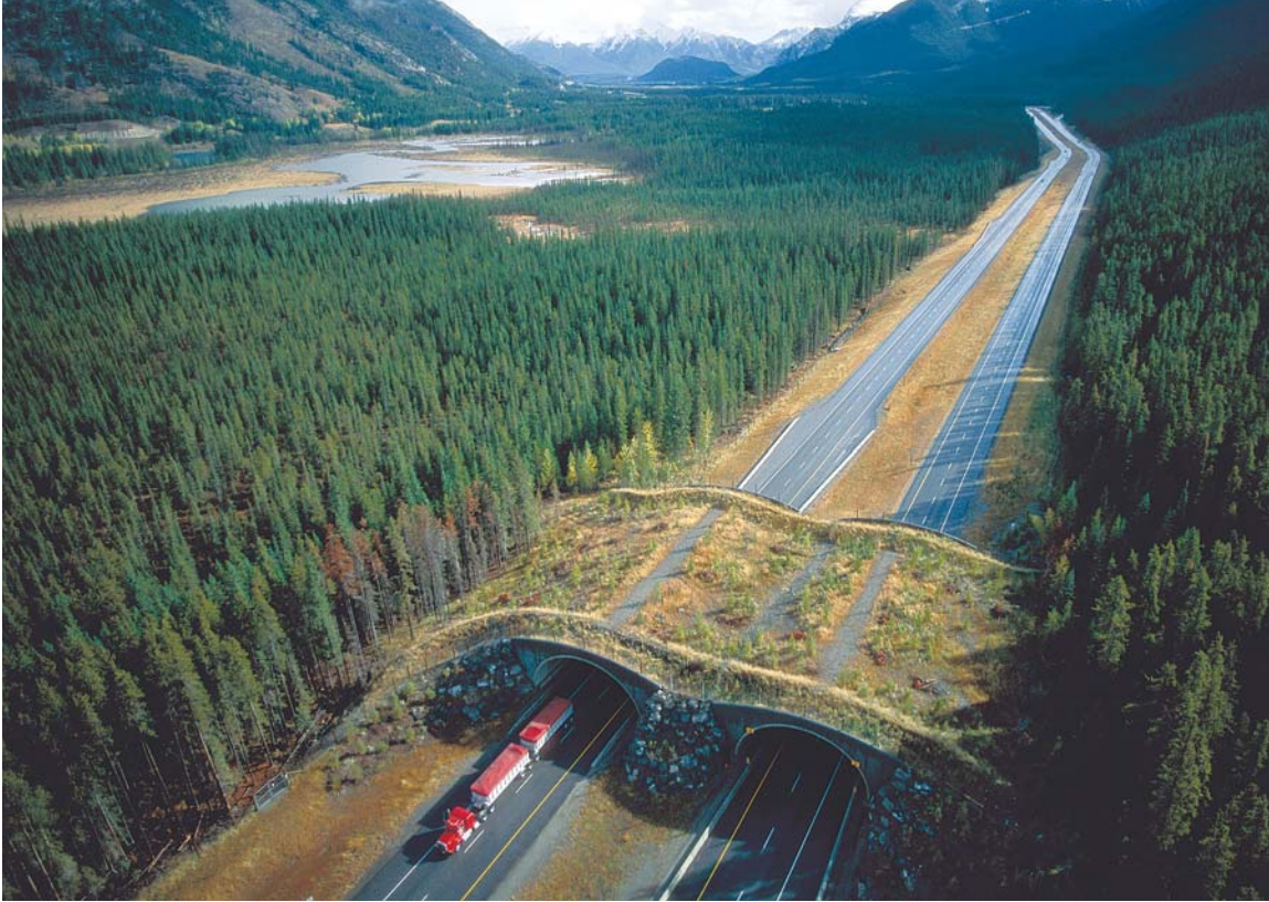
Roads and the vehicles traveling on them pose a significant threat to wildlife. Special road-crossings such as this landscaped overpass near Banff National Park in Alberta, Canada, can help reduce the risk of collisions between drivers and animals.
