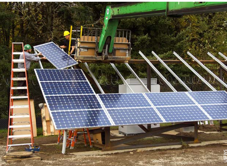
Solar panels under construction.
