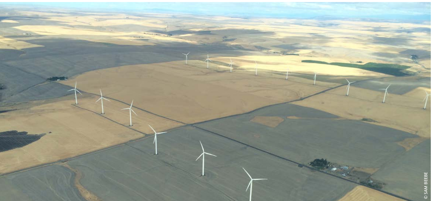
Aerial view of wind turbines in Oregon.
