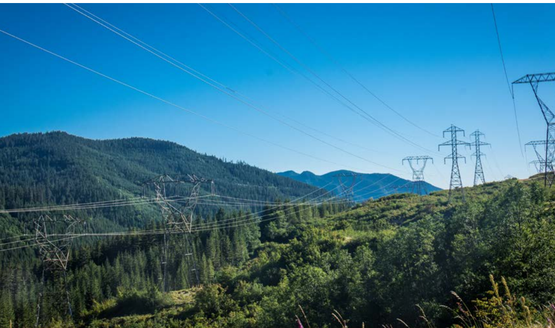
Transmission lines along Lolo Pass in Clackamas County.
