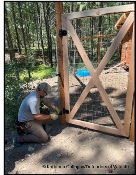
Defenders' Russ Talmo constructing a bear-resistant electric fence to secure a resident's chicken coop.
