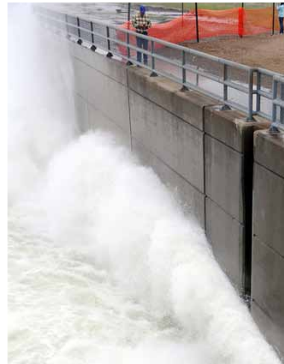
Pent-up floodwaters rush from Oahe Dam in the Missouri River Basin.
