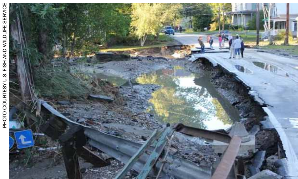
Residents of Bethel, Vt. survey a roadway washed out by flooding caused by the heavy rains of Hurricane Irene in 2011. Linked to damages and losses totalling $9.8 billion, Irene helped make 2011 the stormiest and most costly yet (Fig. 1).
