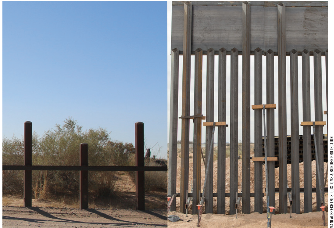
Bollard wall (right) is replacing existing vehicle barriers (left) on the U.S.-Mexico border. (Photos not to scale.)
